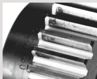
Poor tooth contact and pitting
